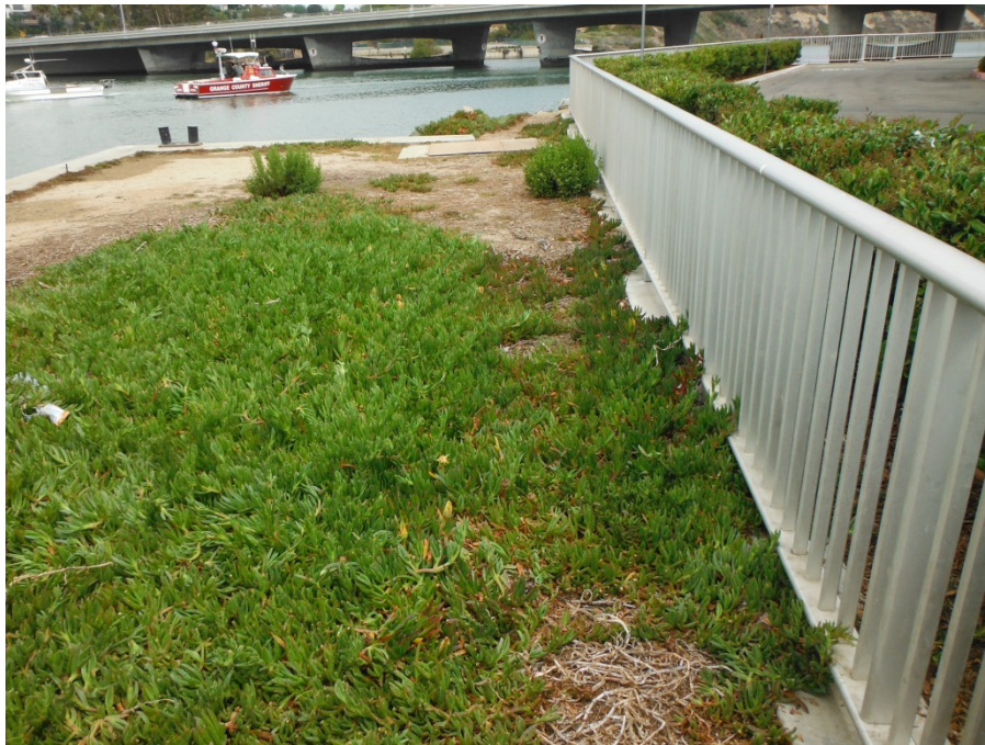
Photograph C-1. Looking north from top of concrete loading platform. The upland parking lot is to the right, and Pacific Coast Highway is to the north.
