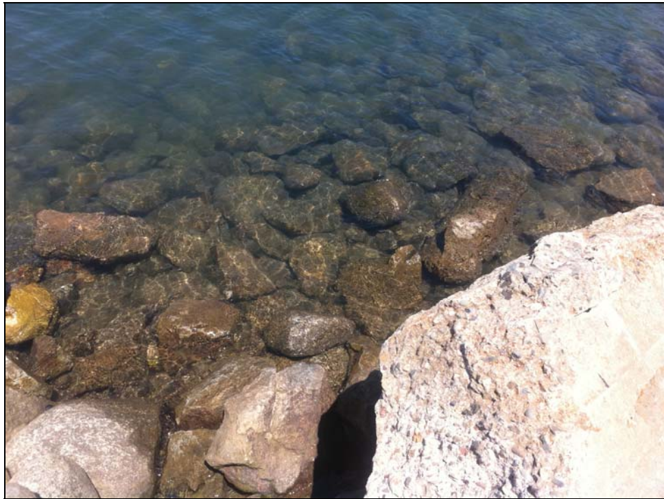
Figure 8. Rip-Rap Along the Shoreline Extending into the Shallow Subtidal Zone
